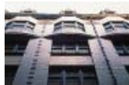
Daily Record Building
